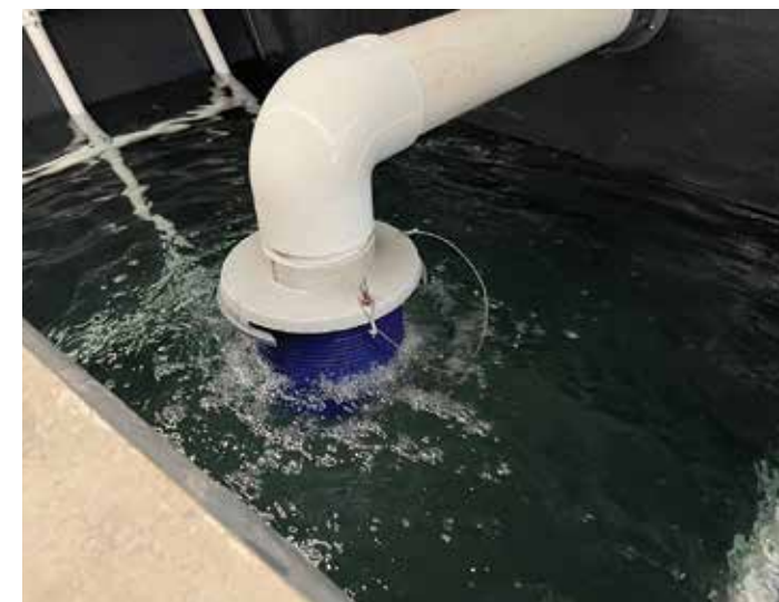
Suspended (above, left) skimmer basket in settlement chamber. Air pumps (above, right) and pond pumps.
