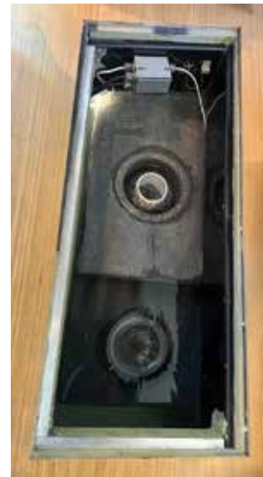
Over-flow regulators under floor with polyurea.
