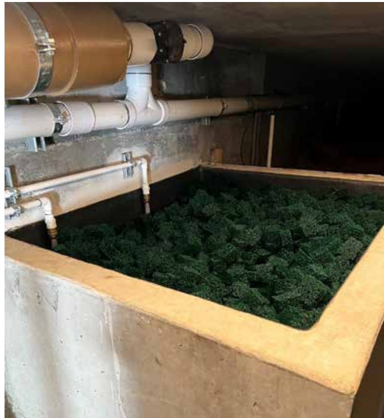
Airated biofilter chamber (top, left) with stainless screens. Aerated chamber (left) with media. Polyurea coating (above) inside tanks.
