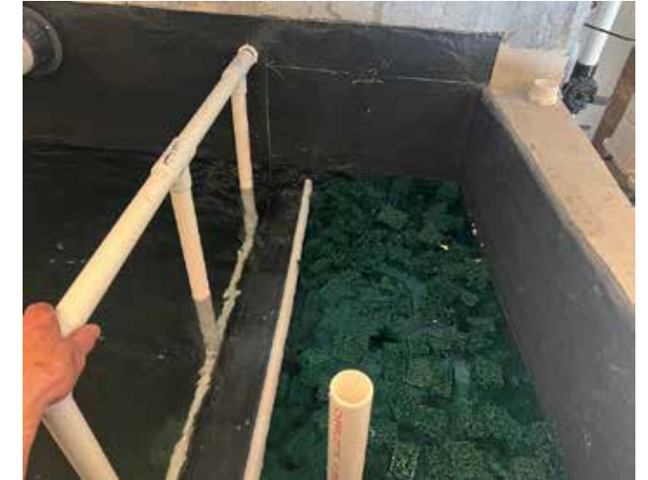
Drains (above, left) in first chamber. Weir plate (above, right) and pre-filter chamber.
