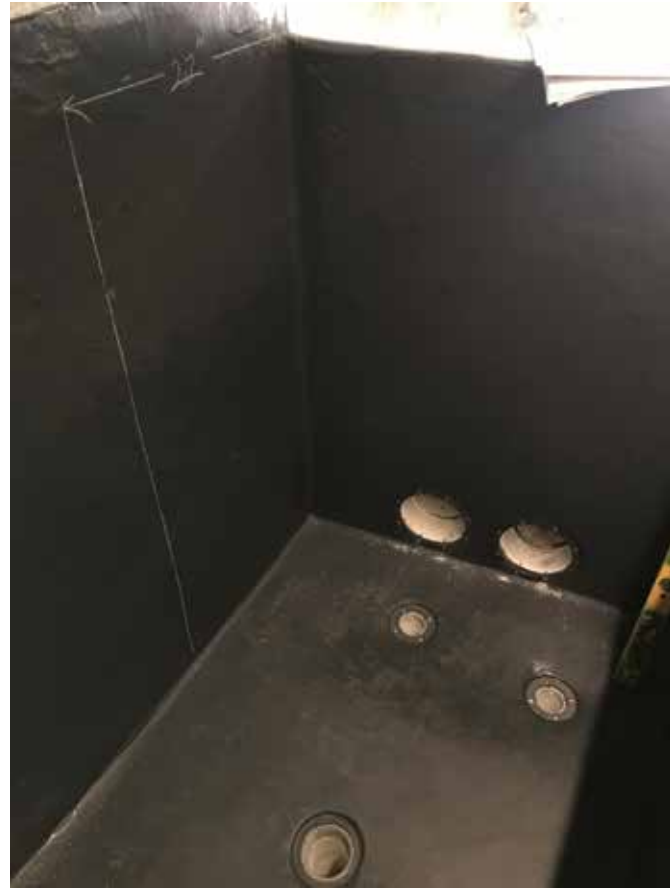
Airated biofilter chamber (top, left) with stainless screens. Aerated chamber (left) with media. Polyurea coating (above) inside tanks.
