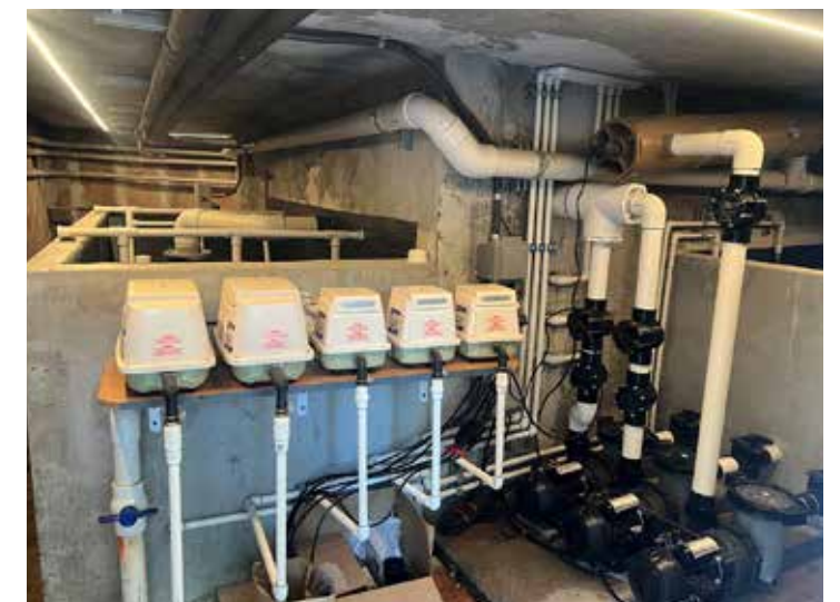
Suspended (above, left) skimmer basket in settlement chamber. Air pumps (above, right) and pond pumps.
