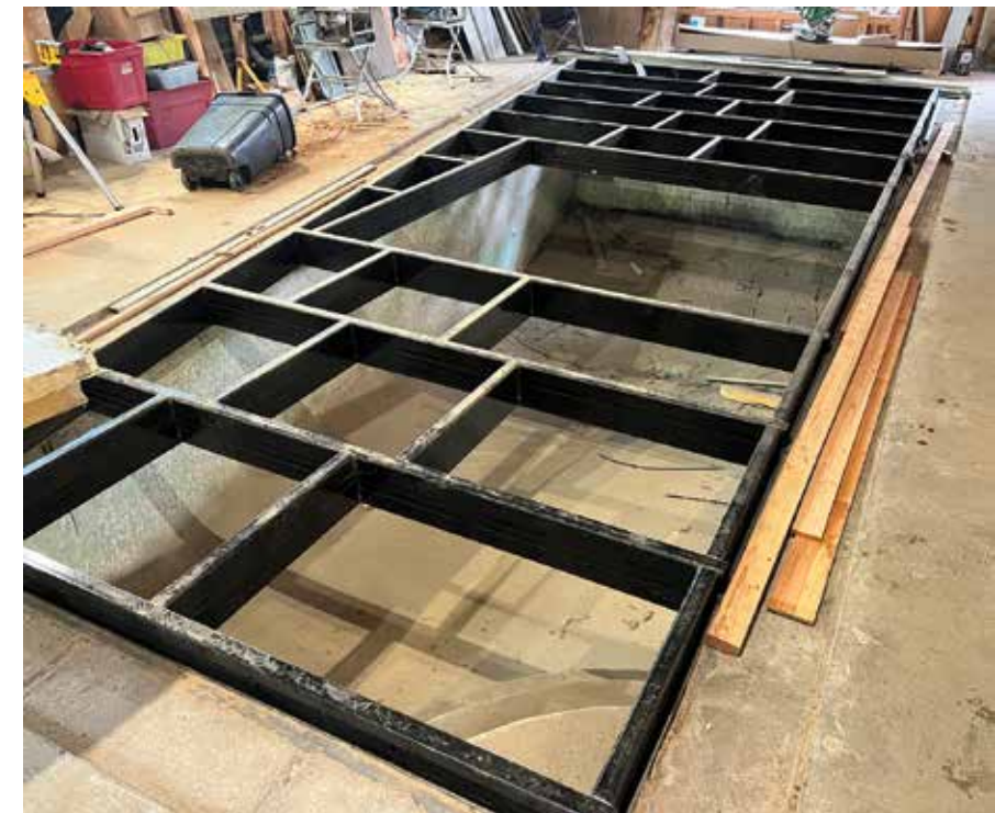
Installation of floor frame.
